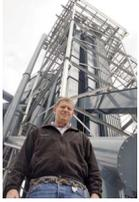
Instead, two legs were installed which contain a grain cleaner and distributor equipped with a computer to direct grain to bins.
